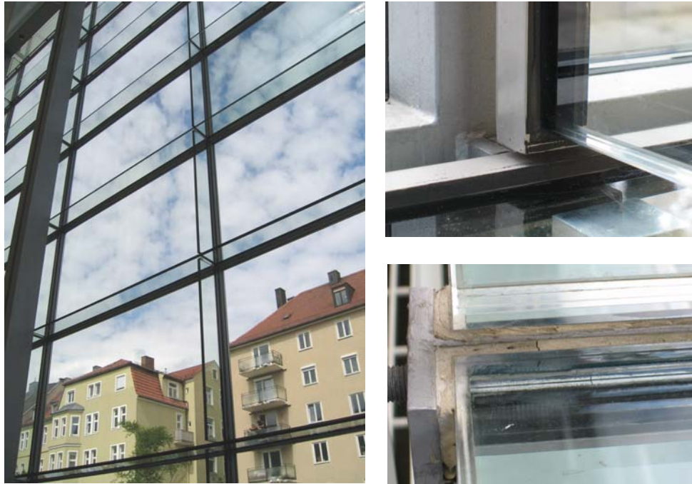
Figure 3 –Glass façade in the year 2008
